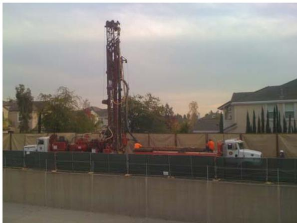
*Pictured above is a drill rig constructing a deep groundwater monitor well along Brea Creek west of the Site.*
