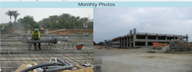
Placing rebar for final deck pour.
